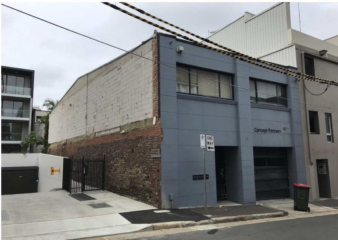
Figure 2: Site as viewed along Brodrick Street.
